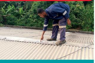
The carpenter carefully points out how the tropical weather has punished the 30-year-old roof which now is badly in need of attention.
